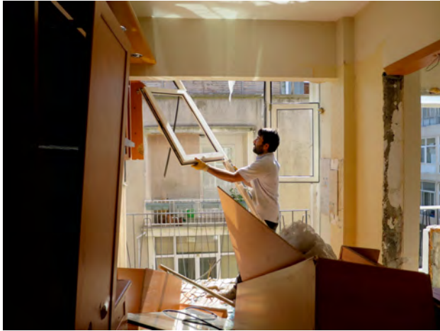
Figure 5.8: Dismantling PVC frames 11
