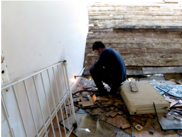
Figure 5.7: Cutting metal pipes 10
